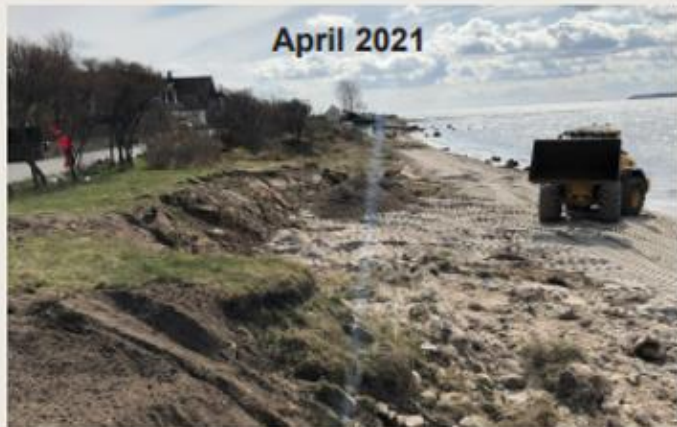
Dunes at Fortuna beach prior to construction.
