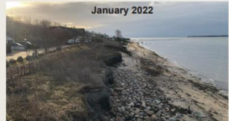
Storm Malik led to significant dune erosion mid-construction.
