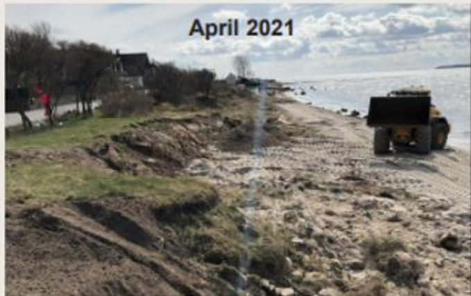
Dunes at Fortuna beach prior to construction.
